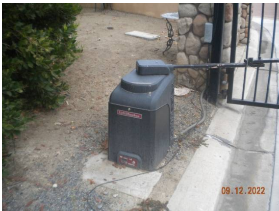
Visual Condition of Complex at the time of Inspection, 09/12/2022
